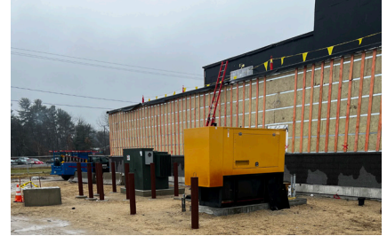
Above: Exterior wall furring at locker rooms.
