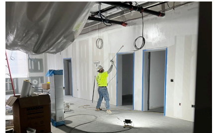
Above: Priming and painting of drywall in new addition.
